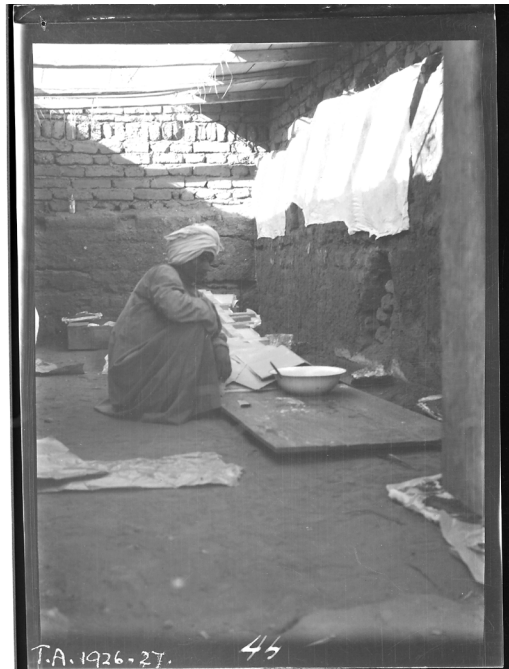
Fig. 8 On site conservation/transfer work at Amarna 1926, facing material is applied to the wall painting fragment to be detached (image courtesy of the Egypt Exploration Society)
